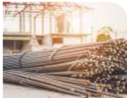
All Civil Material Supply
