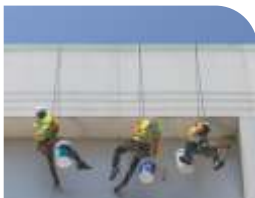
Painting and Coating work
